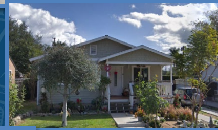
Habitat for Humanity Single Family
