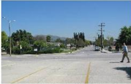
Site entrance at Grand looking east toward Meda Ave. Future signal
