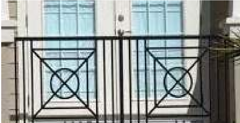
Fixed decorative grillwork and railings are allowed in the Specific Plan area
