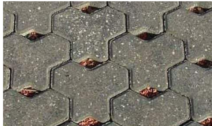
Permeable pavements filter runoff for groundwater recharge
