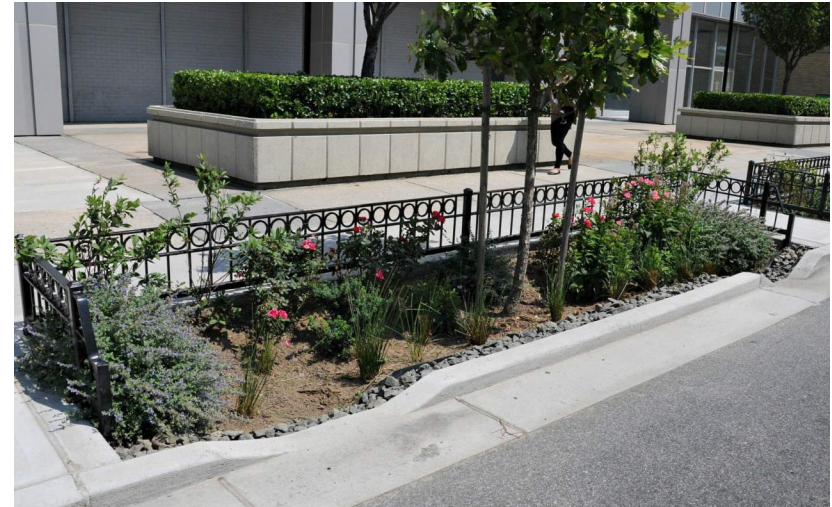
Decorative planters enhance the streetscape and help to clean run off
