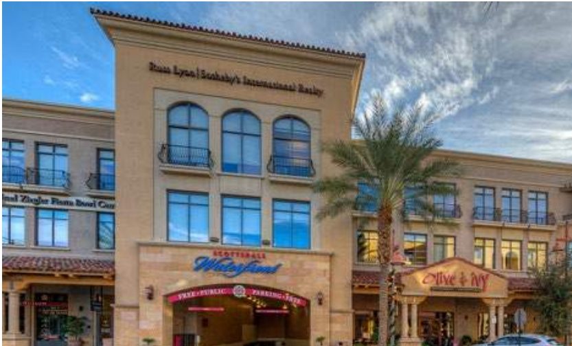
The MU-CC attracts street life with a mix of high density residential and commercial
