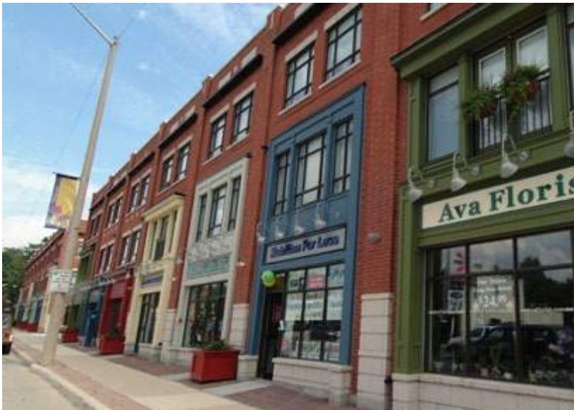
Opportunities for rehabilitating older buildings exist on Arrow Highway
