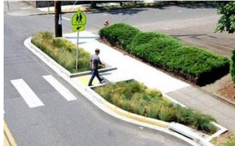
Bulbouts improve safety and visibility of crosswalks
