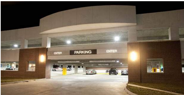
Directional lighting provides visibility and safety for parking structures
