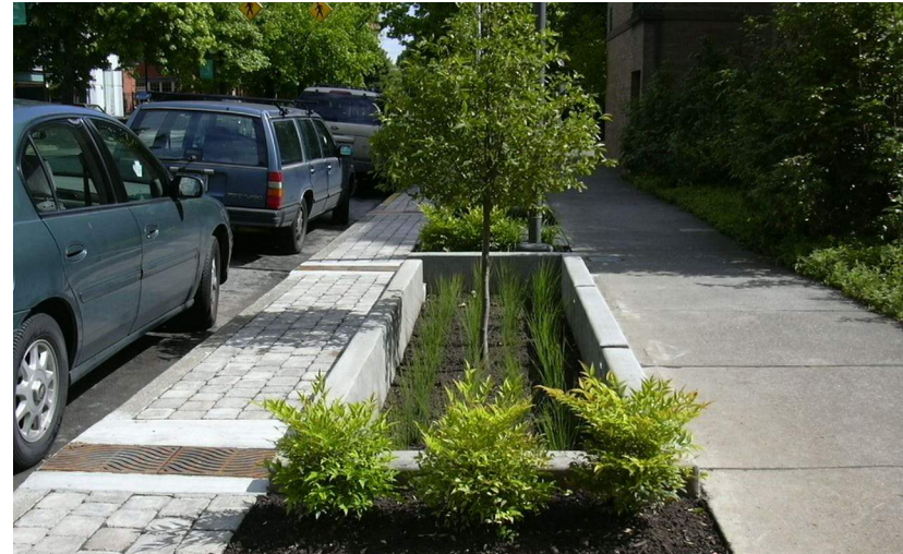
Bioswale planters treat urban runoff while enhancing aesthetics
