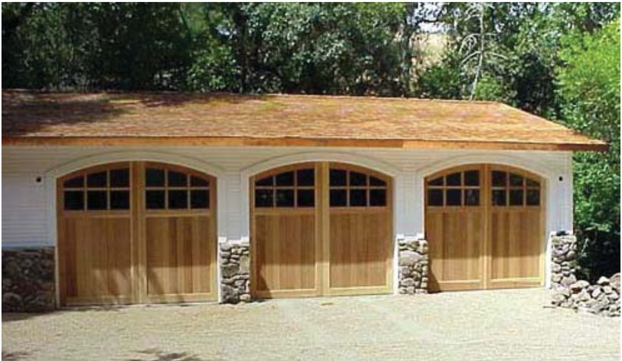
Separate Garage Doors
