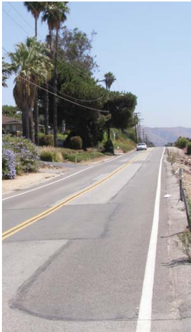
Sierra Madre Avenue will be widened with more defined shoulders and edges, plus the introduction of a safe sidewalk and an improved intersection at Barranca Avenue.
