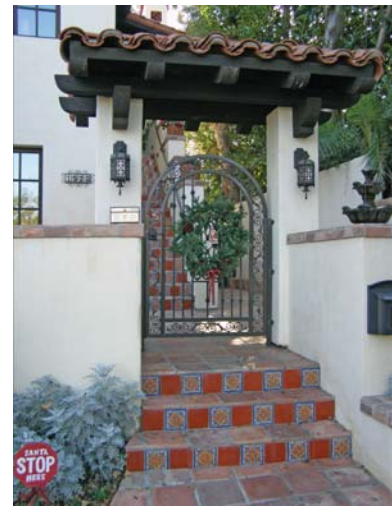
Preferably perimeter walls would extend from an exterior wall of the main building and exhibit identical, or complimentary, exterior color and cladding.
