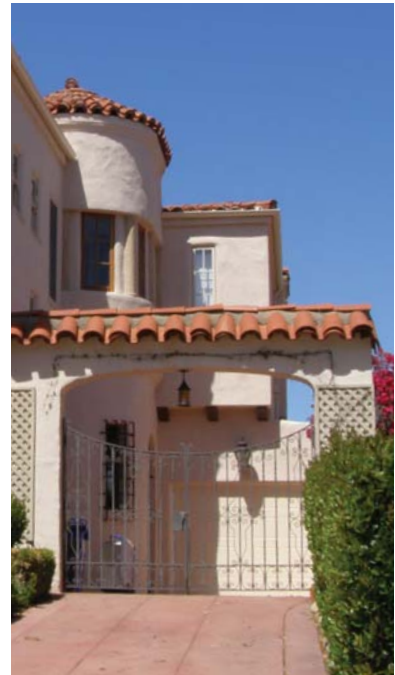
Gate across the driveway behind the front yard setback
