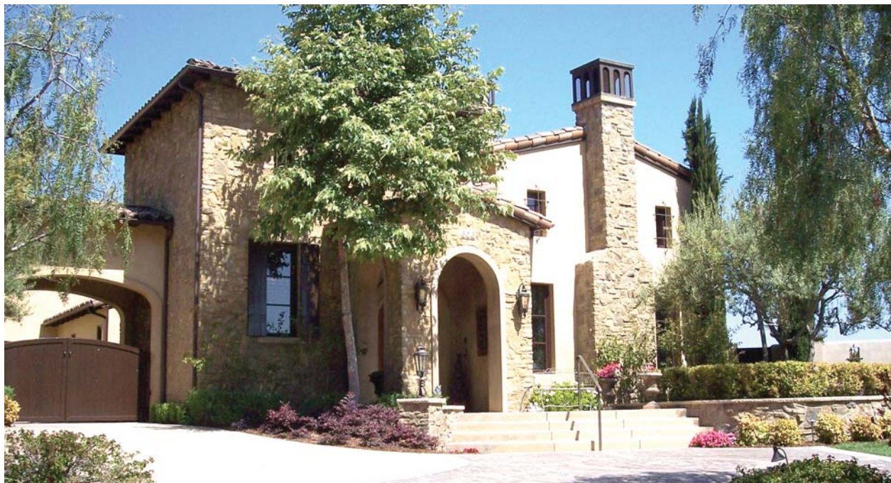
The image (below) is a good example of a balanced mix of exterior wall treatments blending stucco and stone.
