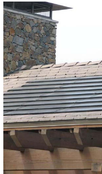
A solar collector (ca. 2010) that resembles roofing material and is less obtrusive
