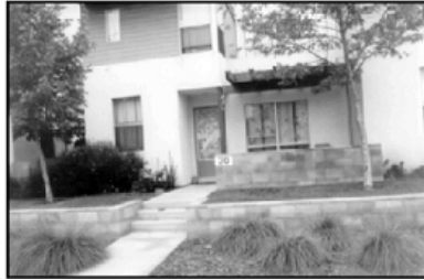
Low retaining walls in the front yard
