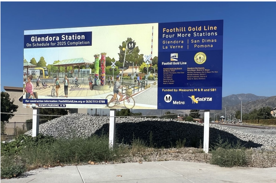
Glendora Station under construction
