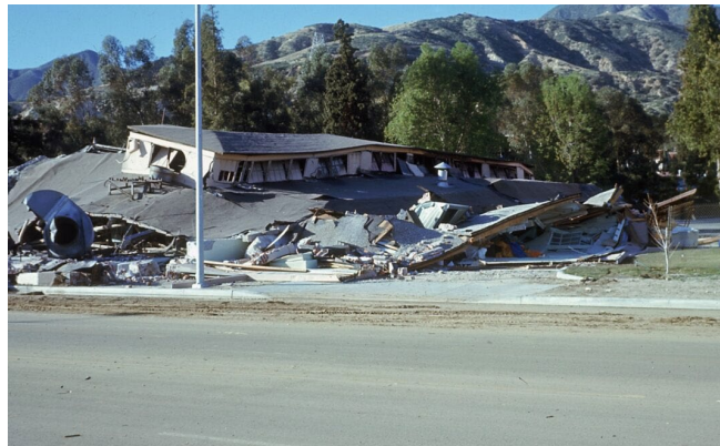
Source: County of Los Angeles Fire Department, Northridge Earthquake 30th Anniversary: Reflections and Lessons Learned , https://fire.lacounty.gov/northridge-earthquake-30th-anniversary-reflections-and-lessons-learned/ , accessed November 21, 2024.
